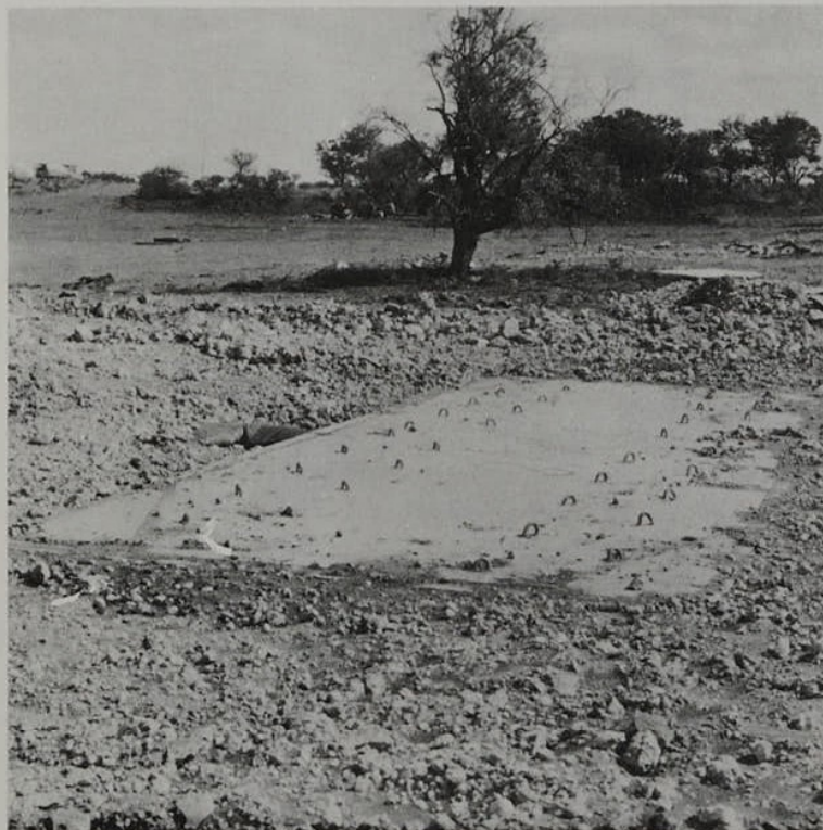
FIG. 9. PANEL IN SURFACE IN POSITION BEFORE ENTRANCE SHAFT SEALED.
